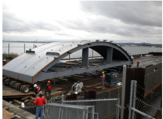
Navigation lock gate sections. Corps photo
